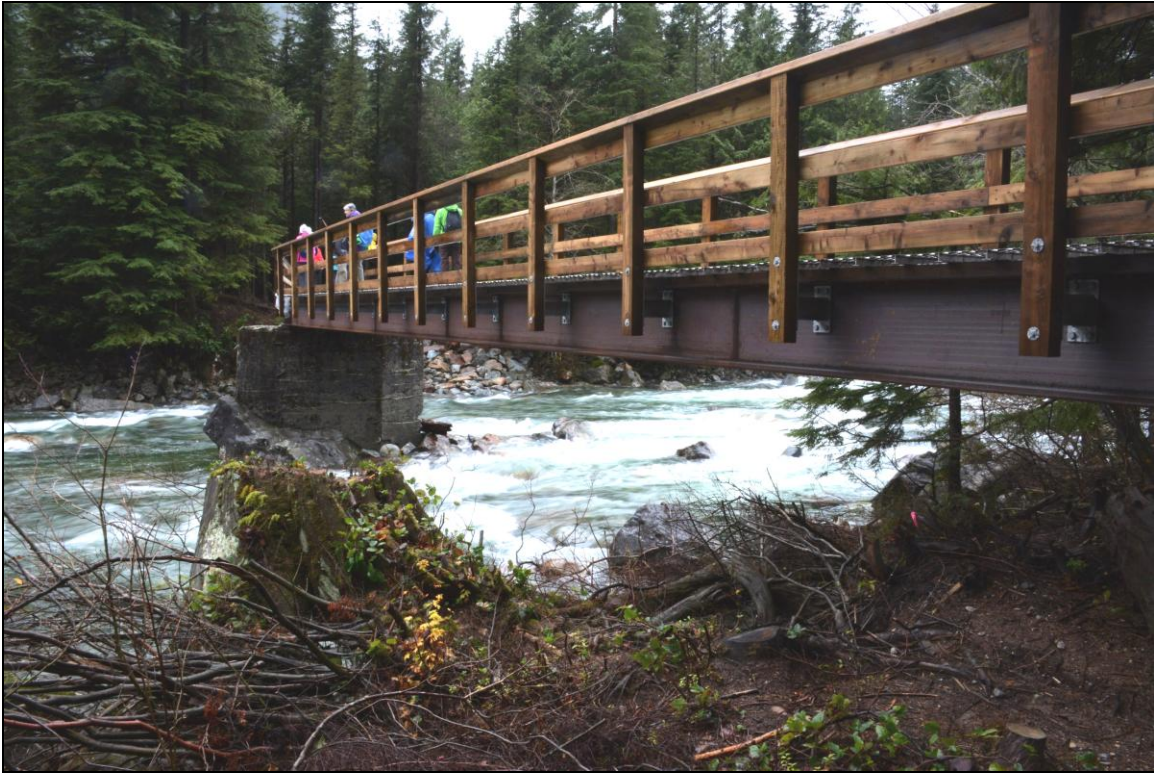
The new bridge over Gold Creek. Ian McArthur photo.
